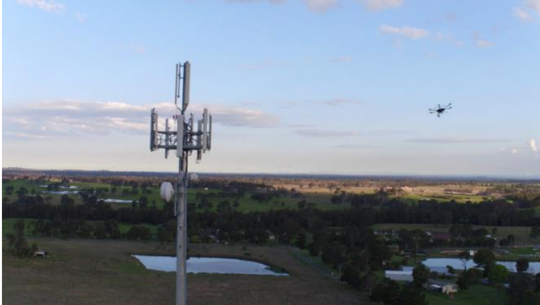
Fig 5.3.7: Cell tower inspection using drone
